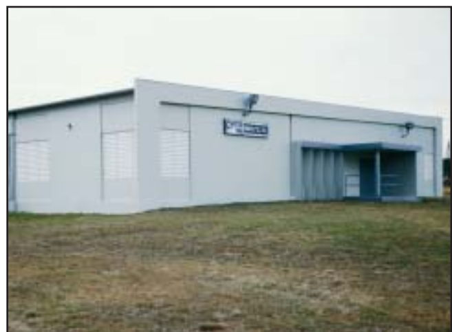
23,500 sq. ft. Fajardo, Puerto Rico facility
